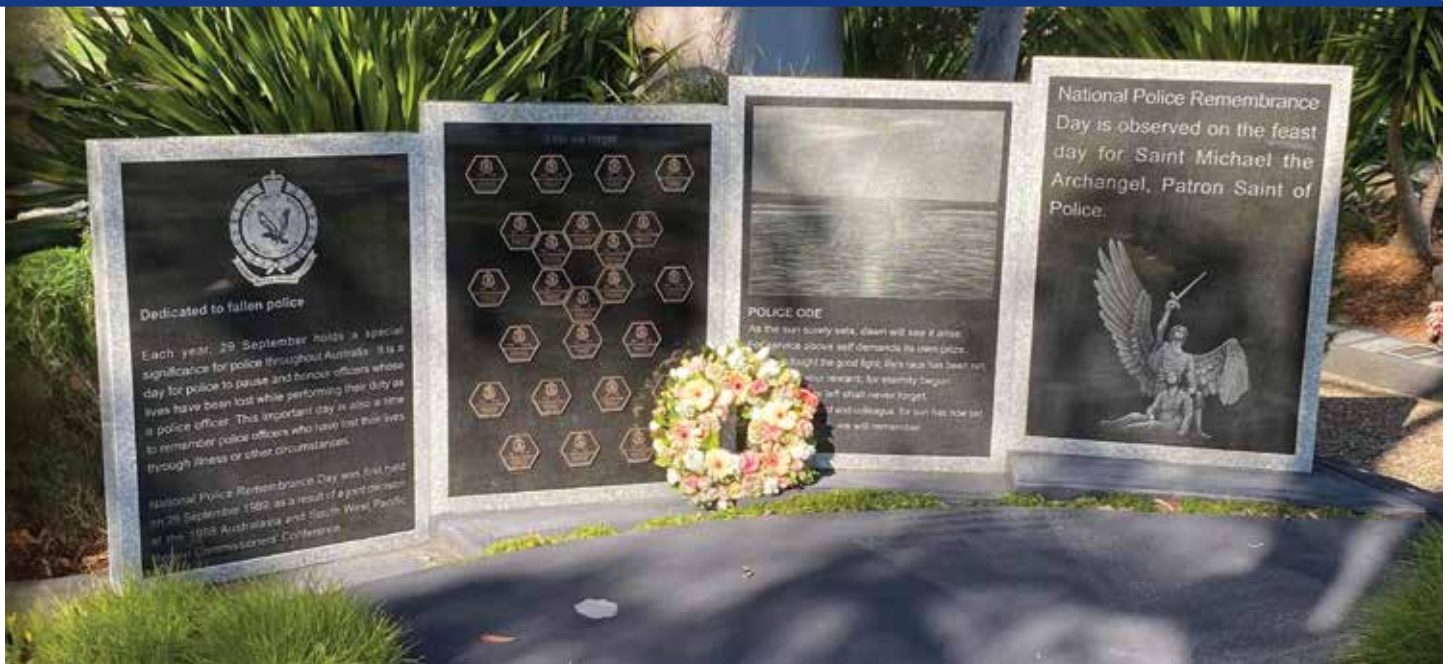
FIRST OF ITS KIND, WORONORA POLICE MEMORIAL WALL, WITHIN WORONORA CEMETERY, WAS COMPLETED IN 2015
